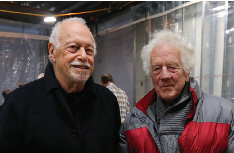
Sansum Clinic Trustee Eddie Rosenblatt with Dr. Virgil Elings in the new Elings Oncology Building (under construction).
